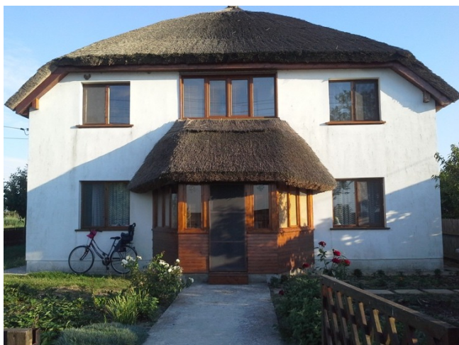
Figure 9. A traditional house in Crișan, Crișan village. The height cannot be more than two floors and the roof must be made of reed or green/blue wood. Photograph: Elitsa Barukchieva, 2015®.
