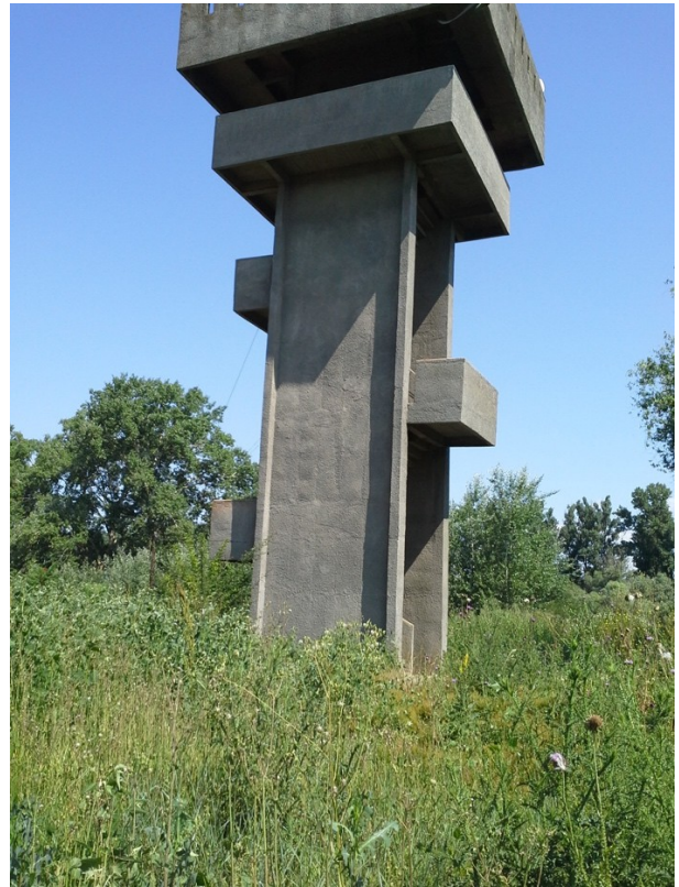
Figure 6. Watchtower, Visitor Information Centre in Crisan. Photograph: Elitsa Barukchieva, 2015.
